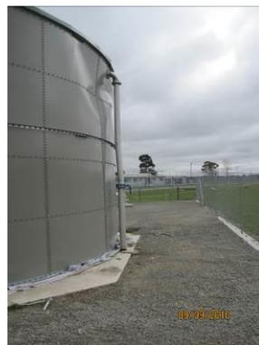
This photograph shows damage caused by rigidly welded pipework entering the top of a tank following the 2010 Christchurch earthquake. This could have probably been avoided if:
