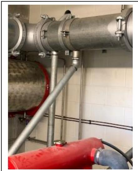
This photograph shows bracing on a 200mm pipe in a pump house.
