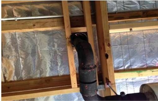
Even minor details such as exhaust runs can be problematic. This exhaust pipe is intimate with the timber framing and is exhibiting signs of pyrolysis.
