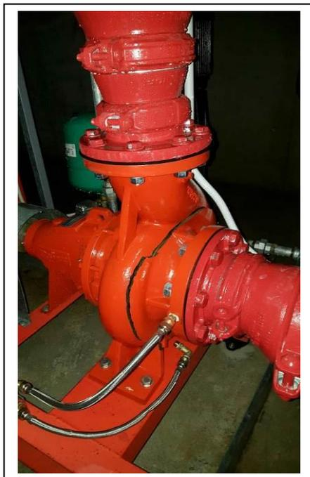
The consequences of getting it wrong can be horrendous. This photograph shows the result of a poorly designed test return, where the butterfly valve failed and slammed shut resulting in water hammer. The water damage from the split pump resulted in a six figure insurance claim.
