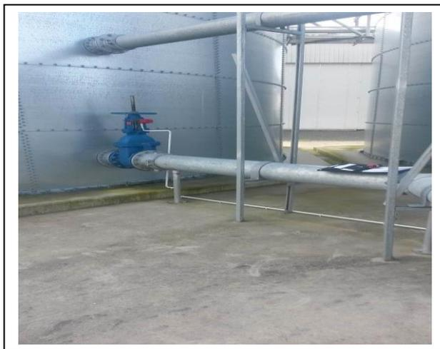
This photograph shows a pipe support which appears to be fabricated out of “Unistrut” type channel.
