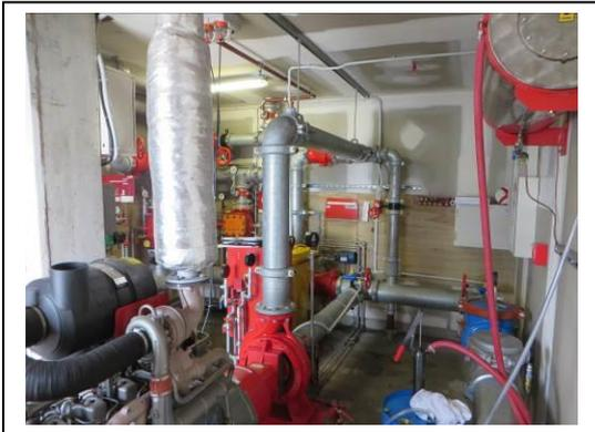
This photograph shows a pump installation of approximately 10 years ago, that was never certified. The issues with bracketing and bracing are numerous to most untrained eyes.
