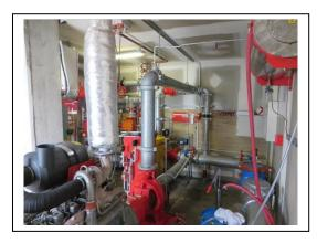
This photograph shows a pump installation of approximately 10 years ago, that was never certified. The issues with bracketing and bracing are numerous to most untrained eyes.
