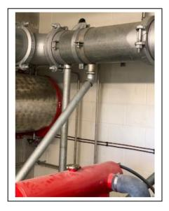
This photograph shows bracing on a 200mm pipe in a pump house.
