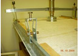
Same squeeze type clip correctly installed
