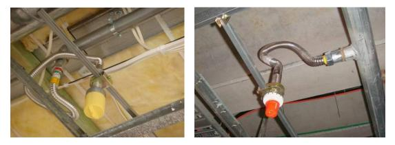
Two examples of over length flexible droppers, with excessive number of bends, or bends not meeting minimum bend radius requirements.
