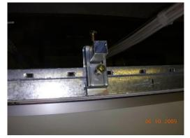
Squeeze type clip incorrectly installed in a clamp style
