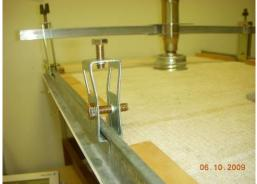
Same squeeze type clip correctly installed
