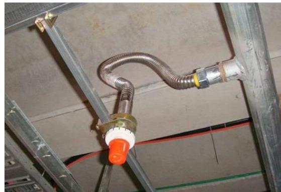
*Two examples of over length flexible droppers, with excessive number of bends, or bends not meeting minimum bend radius requirements.*
