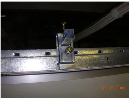
*Squeeze type clip incorrectly installed in a clamp style*
