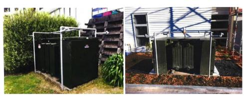
NZS4541:2013 requires that the potential for a fire from an external fire load be prevented from spreading into a sprinkler protected building. There are a number of ways to achieve this:
