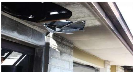
Figure 6: 30 minute fire rated soffit
