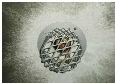
*Guard fitted to sprinkler head in room of fire origin*
