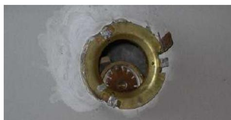
*Recessed sprinkler head in hallway unable to drop down*
