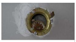
Recessed sprinkler head in hallway unable to drop
