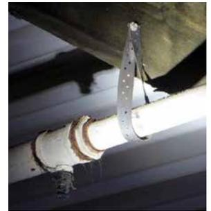
**Flexible droppers are supplied with ceiling brackets for a reason.** Pipe clips and saddles don't grip the dropper properly, as a result the
