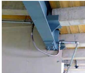
**Flexible dropper used as seismic joint.** There are two problems here. Firstly the losses though flexible droppers are significant; did the designer build those into their design? Secondly flexible dropper are only designed and tested for
