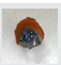
Smoke can spread through poorly installed fire stopping systems like in the photo below which had a real fire on the other side of the plasterboard wall. While this may seem insignificant to some, with many penetrations like this, they will allow considerable amount of smoke through to another fire cell. If this is a rest home or hospital then it is even more critical.
