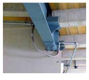
Flexible dropper used as seismic joint. There are two problems here. Firstly the losses though flexible droppers are significant; did the designer build those into their design? Secondly flexible dropper are only designed and tested for
