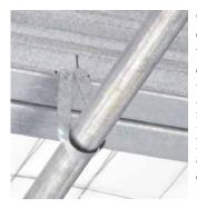
Over size twist clip. This clip is one size bigger than the pipe. As a result the clip is not tightly holding the pipe. This means the pipe is no longer restrained longitudinally and potentially may shift. Same also applies when pipe clips aren't the correct size.
