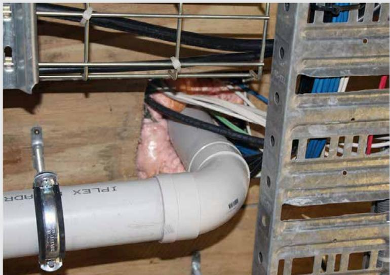
*This is a timber infill type floor with concrete above the wood. The foam may be the right depth however is not the correct system for the cables and PVC pipe.*
