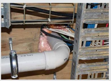
This is a timber infill type floor with concrete above the wood. The foam may be the right depth however is not the correct system for the cables and PVC pipe.
