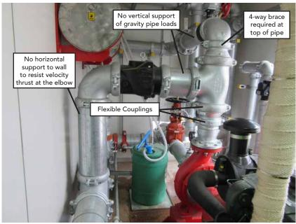
of the pipe thread. It is worthwhile borrowing from the petrochemical sector where they use RHS or C channel as the post, or the mechanical services sector who build pipe ladders from pre-engineered metal framing systems; when of sufficient size such materials afford lateral and longitudinal bracing as well.
