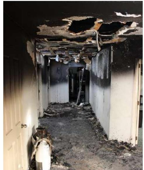
Photo above shows extensive fire damage in first unit.
