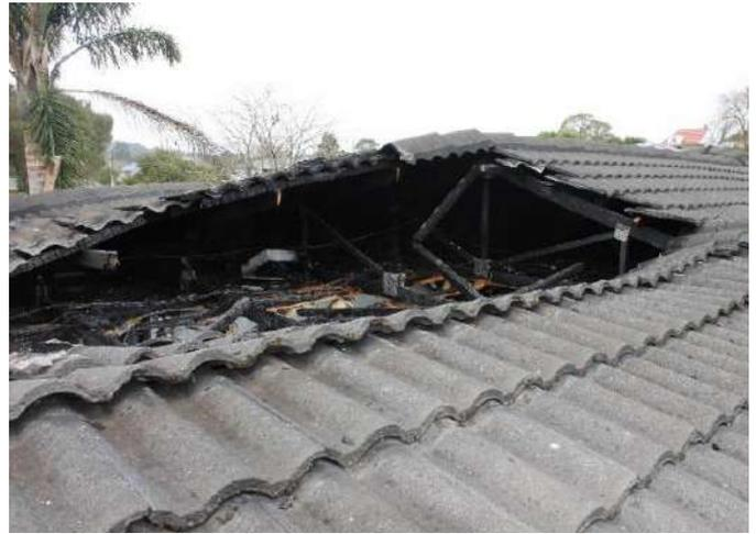
Image above shows partial roof collapse on the fire side of the separation wall.
