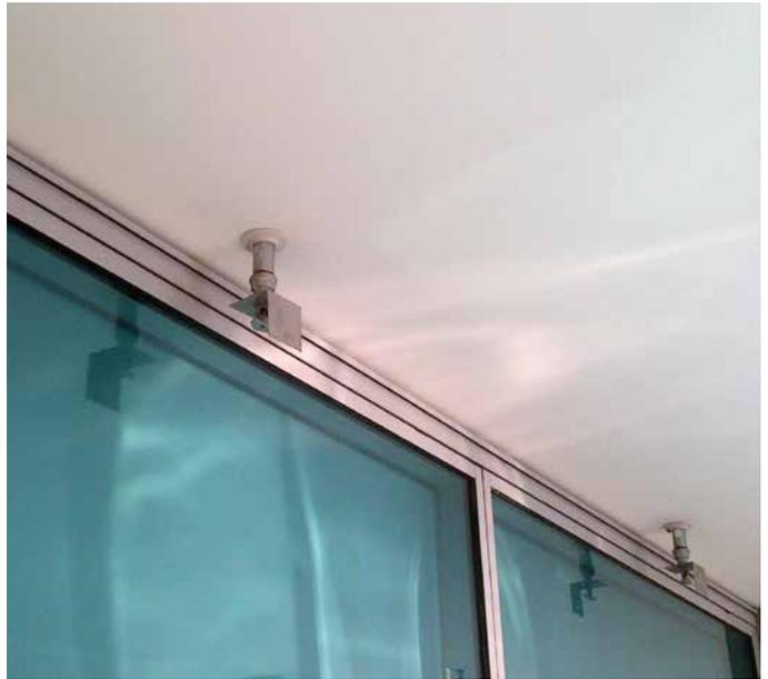
On face value, this installation appears sound, albeit, some form of unapproved baffle plates have been fitted to both window sprinklers.
