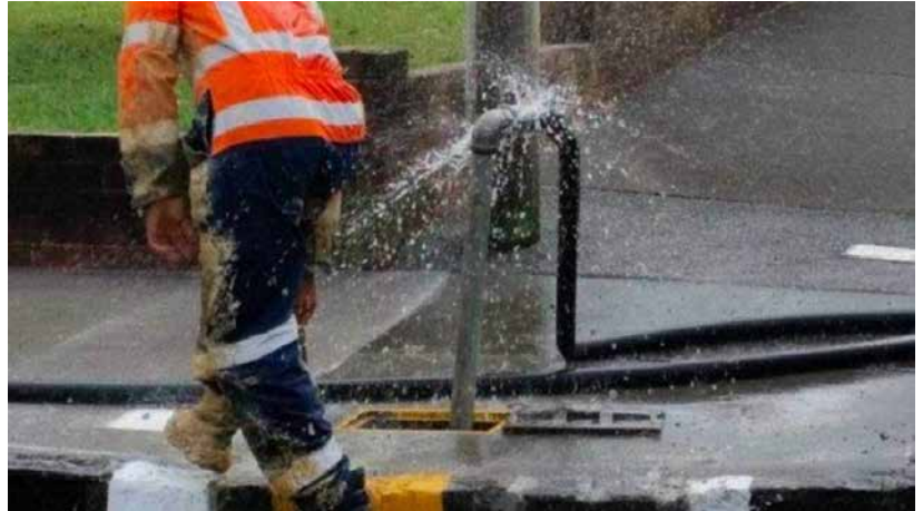
An unauthorised connection to Auckland's water network using an unapproved standpipe.
