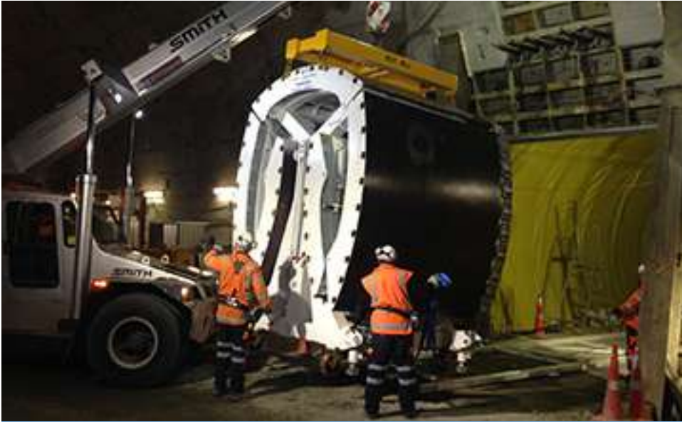
20t crane lifting the arch form onto the steel track.
