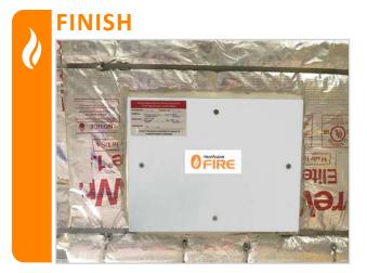
Finish the installation with a fillet of FyreFLEX Sealant to the perimeter of the FyreWrap® Access Panel, ensuring that none of the metal frame remains exposed.
