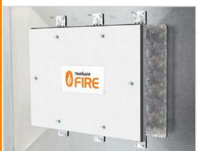
Using the preformed holes in the FWAP frame, drill and fix (using steel rivets or self-tapping screws only) the frame to the ductwork.
