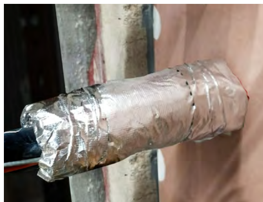
TWRAP™ secured on each side of penetration using three strips of reinforced aluminium tape applied around the wrap's circumference. TWRAP™ applied on both sides of the wall. Alternatively, apply steel ties 50mm from each end and at 150mm centres in between.
