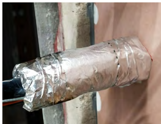
TWRAP TM secured on each side of penetration using three strips of reinforced aluminium tape applied around the wrap's circumference. TWRAP TM applied on both sides of the wall. Alternatively, apply steel ties 50mm from each end and at 150mm centres in between.
