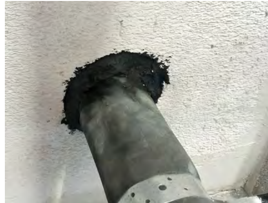
FyrePEX TM HP Sealant applied to a depth of at least 26mm from each side of the wall.
