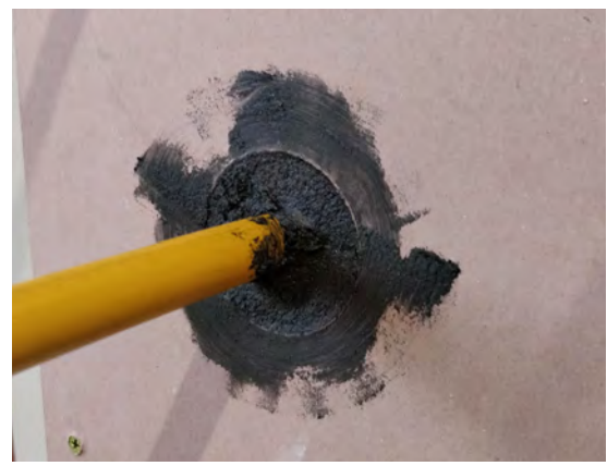
FyrePEX™ HP Sealant filled to the full depth of the plasterboard on both sides of the wall.
