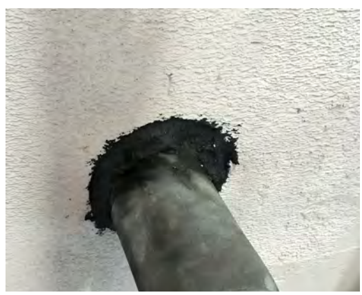
FyrePEX TM HP Sealant applied to a depth of at least 26mm from each side of the wall.
