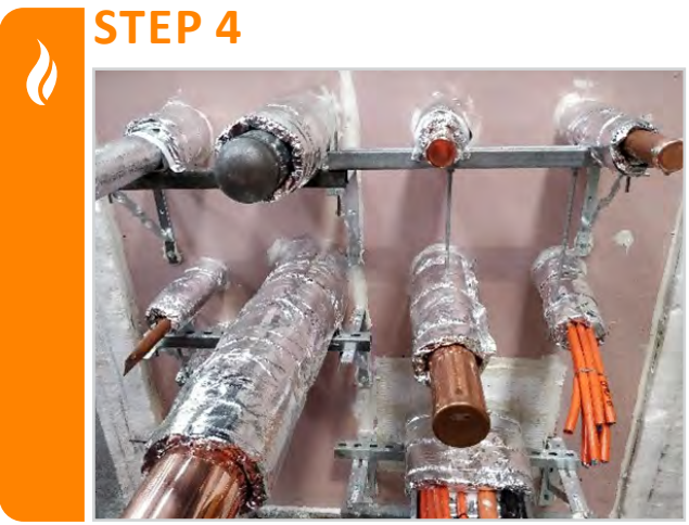
Wrap to the approved length (as per the tables on page 14-15 ) ensuring that where the wrap meets itself, there is a 50mm overlap. Close and cut edges of the wrap with aluminum foil tape and secure wrap to service with steel cable ties. See page 24-26 for technical drawings.
