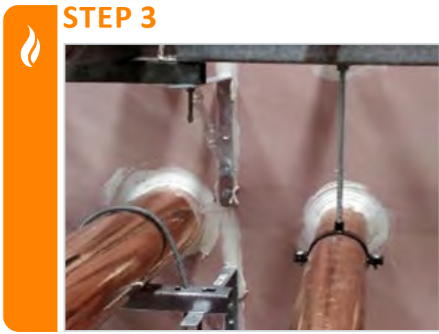
Apply FyreFLEX® Sealant to the full thickness of the plasterboard, ensuring the correct size of fillet (or cone). Sealant needs to be applied to both sides of a wall penetration.
