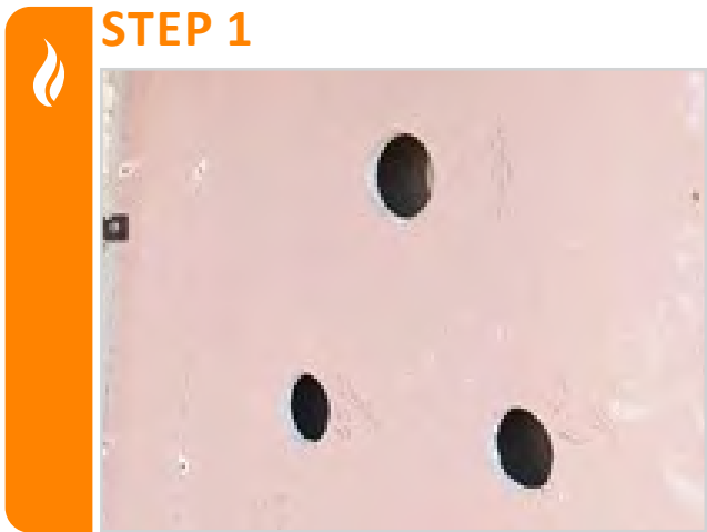
Form an opening appropriate for your service as per the approvals table on page 14-15 . Maintain 50mm between openings if multiple pipes are present.
