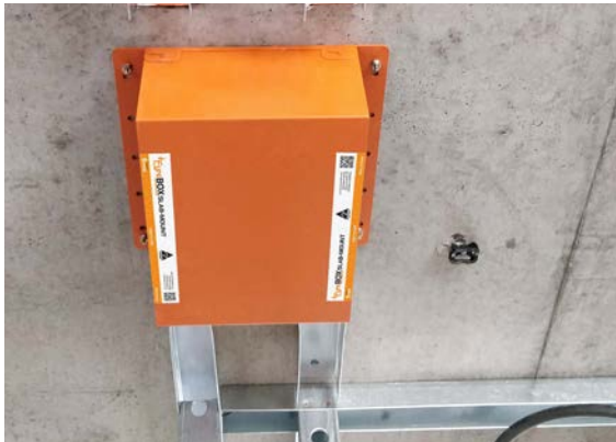
FyreBOX top plate, body and approved services all installed as standard to the soffit, with foam end plugs installed around the services.
