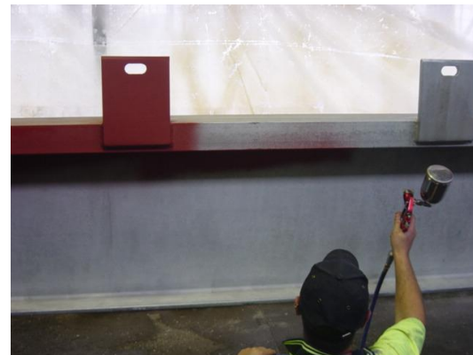
Figure 23 Application of anti-corrosive primer
