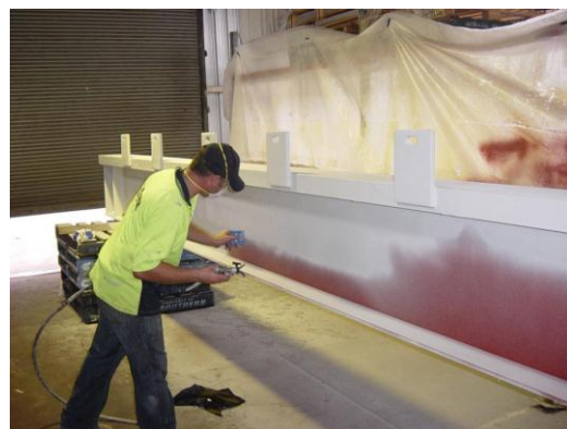
Figure 27 Measuring wet film thickness of intumescent coating
