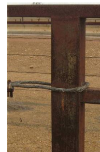
Figure 19 Steel surface pre-blast
