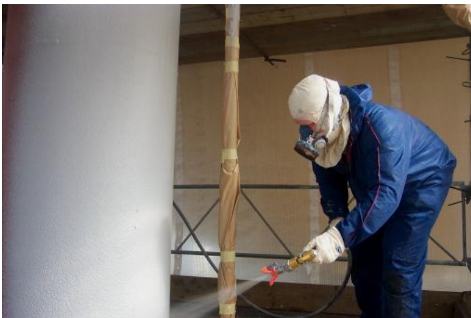
Figure 21 Example of masking to avoid overspray onto other surfaces
