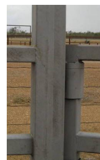
Figure 20 Steel surface after blasting
