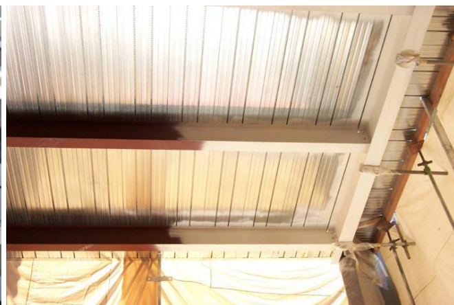
Figure 5 ICS applied to steel beams
