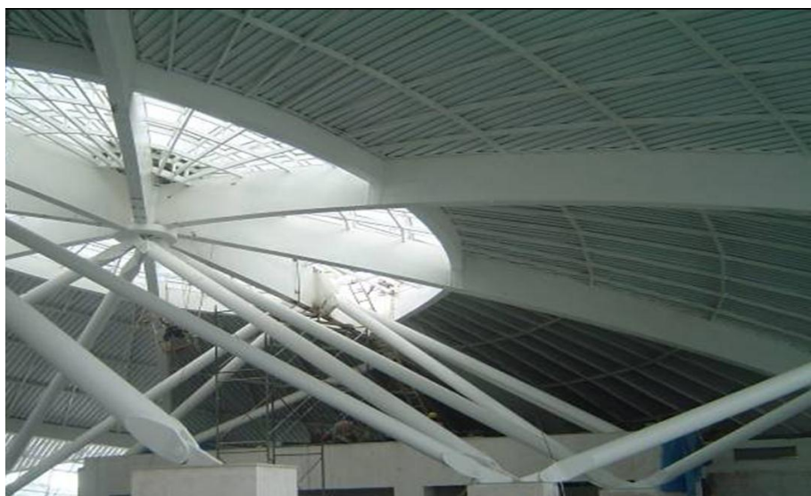
Figure 1 Sample of structural steel with an intumescent coating system applied.
