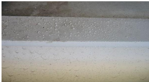
Figure 10 ICS failure - bubbling
