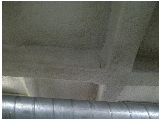
Figure 3 Vermiculite coating on steel beams and slab
