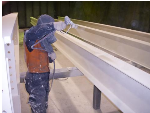
Figure 14 Application of basecoat by spraying
