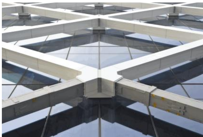
Figure 4 Board product applied to steel beams and columns
