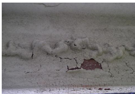
Figure 12 ICS failure – incompatible primer
