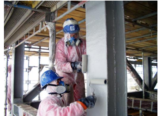
Figure 15 Application of basecoat by roller
