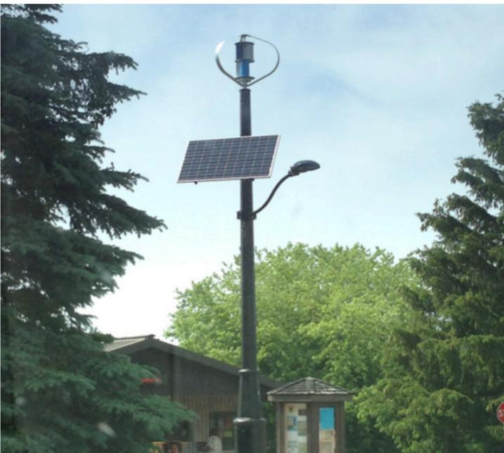
The Earl Rowe light configuration includes a concrete StressCrete pole, a 55W LED street light complete with dimming, a single solar panel, a wind turbine and four 12V batteries.
