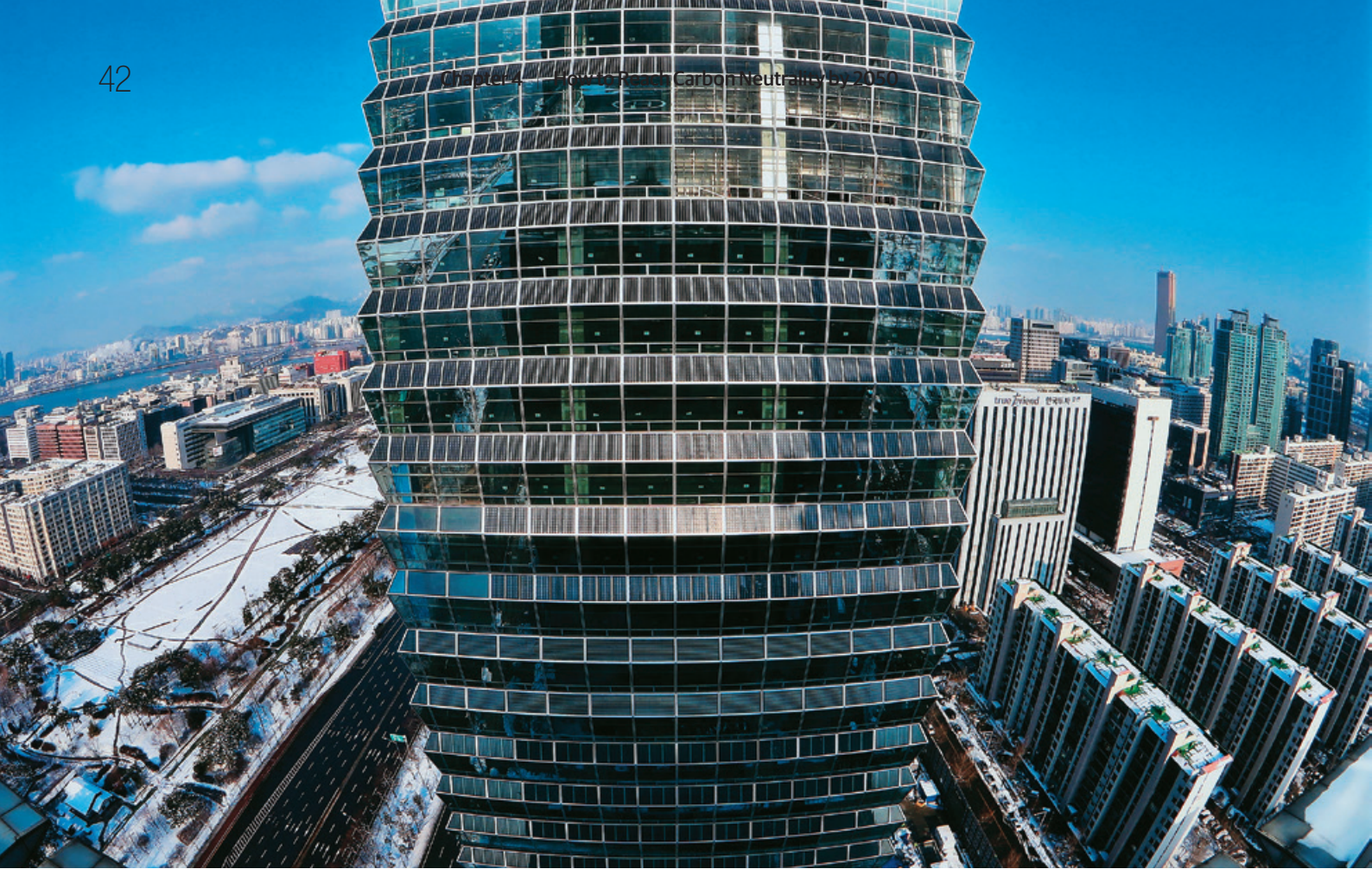
BIPVs used in FKI (Federation of Korean Industries) Tower.
