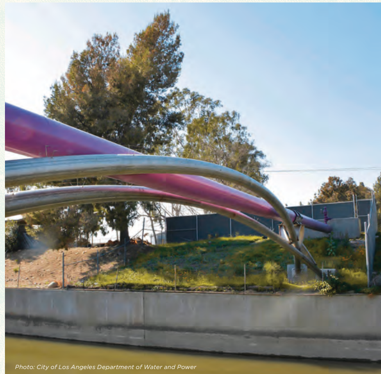
Photo: City of Los Angeles Department of Water and Power
